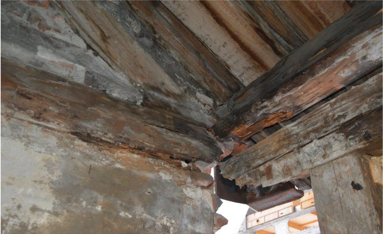
02 Enormous structural damage to all of the geometric envelopes of the 175-year-old residential house at Smedbakken 5 about 40 years after the micro-meteorological reversal of the vapour permeability and the dew point. (Source: Author)
