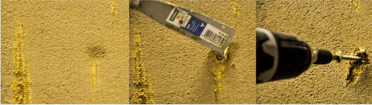
04 Sequence of the dismantling process of earth dry lining boards
