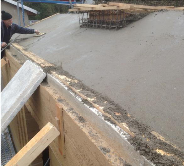
The gable walls had to end in an incline corresponding to the pitch of the roof so that the wall crown can bear the load of the massive earth panels. And this was the next lesson we learned.
