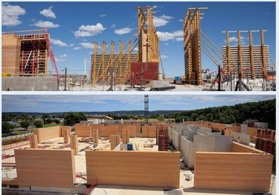
Figure 2. Rammed earth construction and formworks (source : <http://sirewall.com>)
